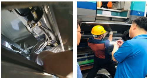
Fig 8 Door step valve and related parts replacement
